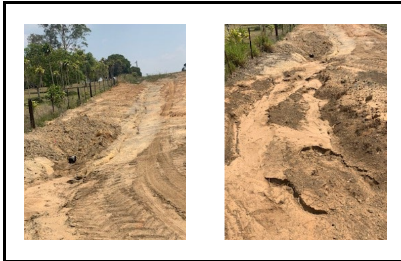
Figure 12: Bioreactor site: Bioreactor after set up (left) and erosion after first rainfall (right).
