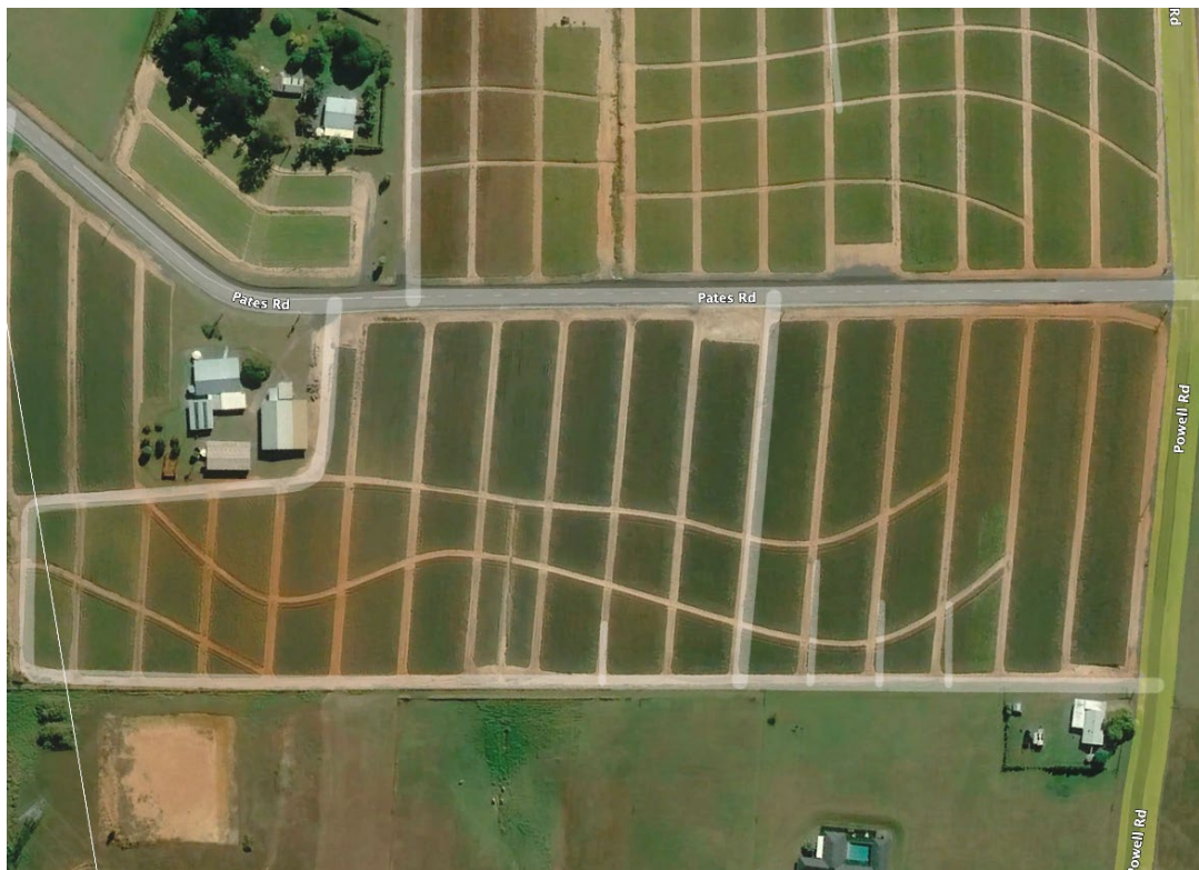
Figure 3: Satellite image of the Pates Road farm after construction of contour drains.
