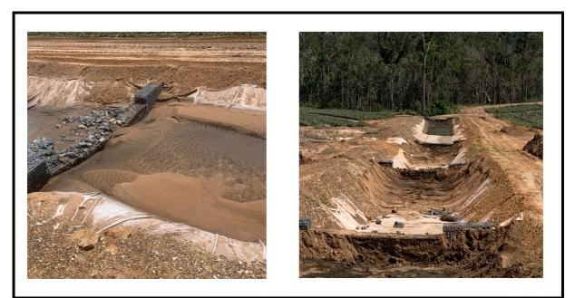
Figure 9: Treatment 2B - Sediment captured behind levy bank (left). Sediment removed from primary drain (right).
